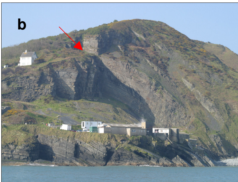
Figure 2.10. Visual survey platforms. a. Mwnt. b. New Quay
